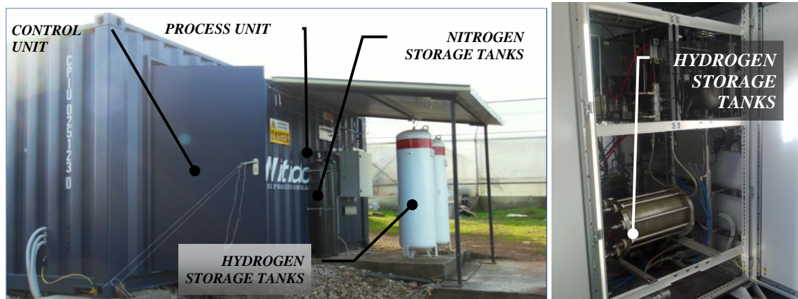
Fig. 1. Stand-alone hydrogen plant external layout and electrolyzer internal stack.
